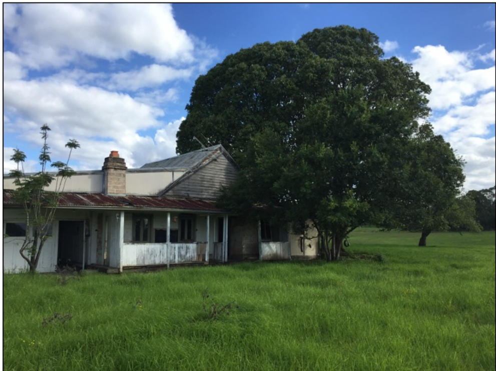
Figure 8. The cottage viewed from the silo.
