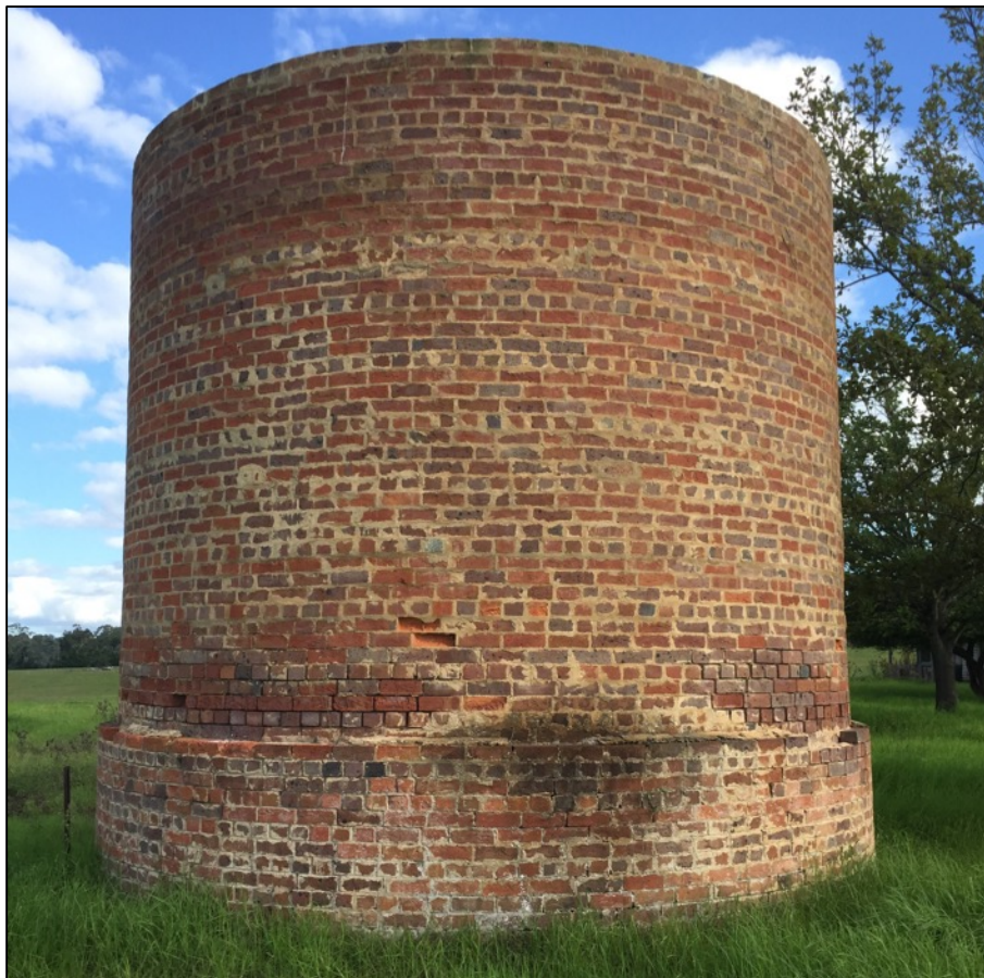
Figure 12: A detail of the brick silo.
