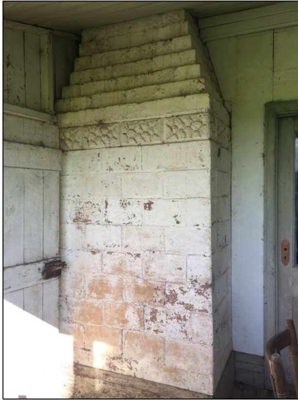
Figure 9. Detail of the middle chimney.
