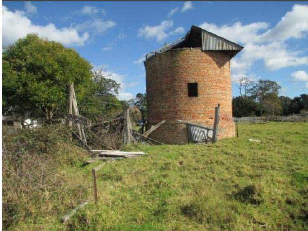
Figure 18: A photograph taken in 2015 shows the gabled roof over the brick silo.
