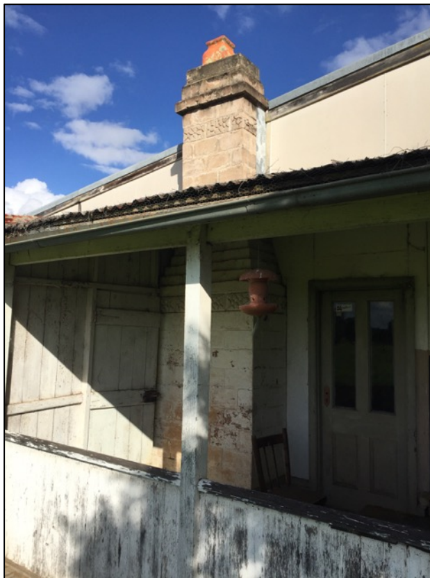
Figure 10. Upper part of the middle chimney.
